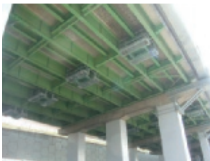
高架橋制振装置 Elevated bridge vibration reduction device
